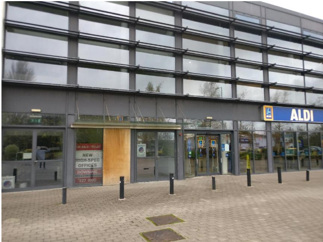
Fig. 3.12. Entrance to Aldi, beside vacant unit
